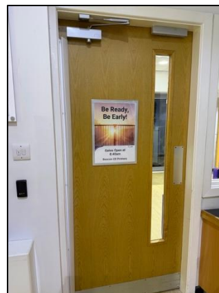
Internal main door at reception
